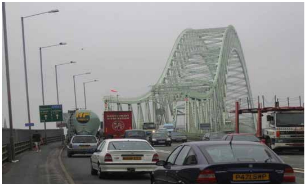
Figure 3.1 – Silver Jubilee Bridge
